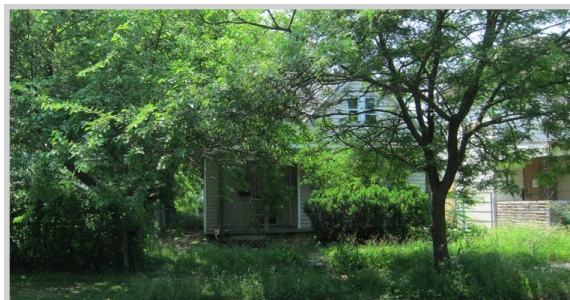
1607 Myrtle Ave. in Linden—one of the properties owned by Start Linden LLC. Code citations included an unsecure building, high grass, and multiple other violations.
